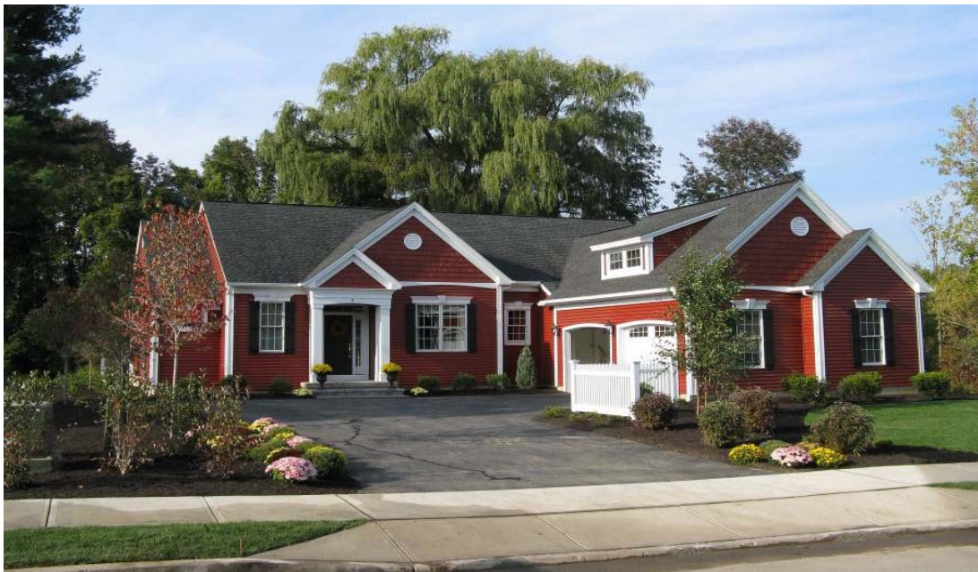
This insulated vinyl sided home by Belmonte Builders pursued LEED® certification and became the first home in the Capital Region of New York to achieve a LEED for Homes' Gold rating.
