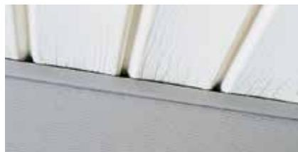
*Ordinary soffit lacks stiffness, so it tends to cup when installed.*
