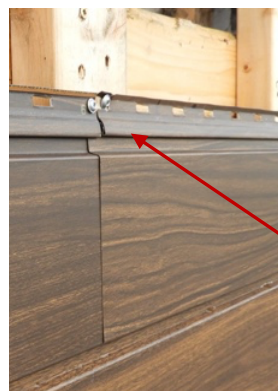
Joint with 2 screws
